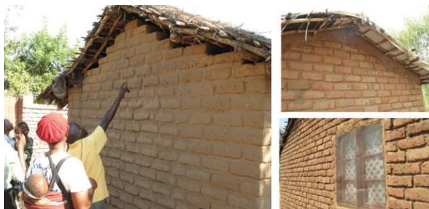
Fig. 2.11. House improvement: community members closing eaves and screening windows in Malawi
