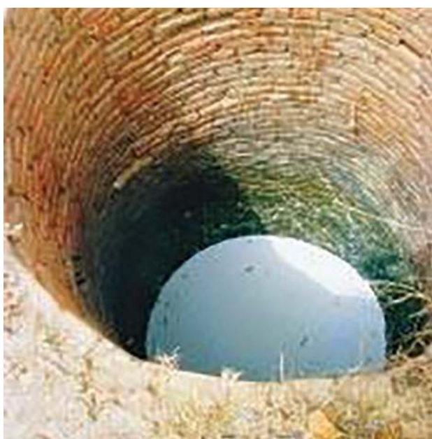
Fig. 2.12. A layer of polystyrene beads prevents mosquito larvae from reaching the water surface to breathe.
